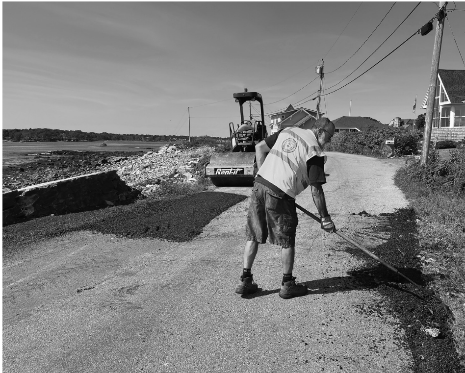
Warren Hathaway City employee Mario Proia patches a section of Seashore Avenue with fresh asphalt on Sept. 11. The project, which included several sections of roadway that were washed out by the January 2024 storms, was completed late this summer. The patchwork is a temporary solution to “get us through the winter,” said Bill Patnaude, the city’s liaison to the islands. Permanent fixes, along with the replacement of a seawall, will be done “sometime between next spring and fall.”
